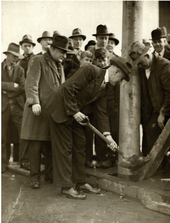
Erecting the first pole 1936 (Port Phillip City Collection sm1744)
