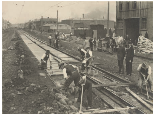
Tramway construction, Sturt Street, 1925 (SLV)
