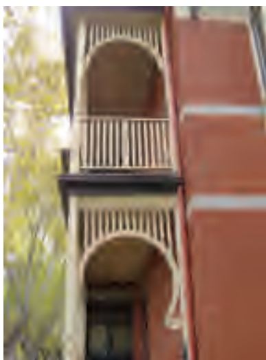
Fig. 1. Simple square balusters and Art Nouveau influenced bracket, with two-dimensional fretwork balusters.
