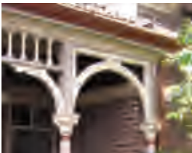
Fig. 4. Cast iron Corinthian capital attached to wood post, with turned balusters on frieze.
