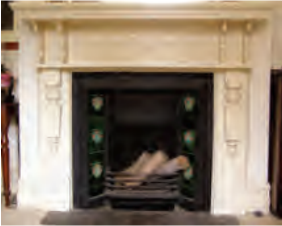
Fig 9. Wood fireplace surround.
