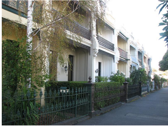
Figure 6.33–7 – A particularly fine row of double-storey rendered terrace houses in Montague Street
