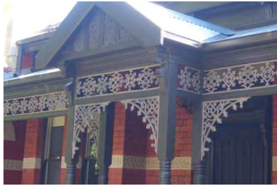
Cast iron encased in wood
