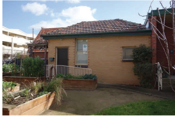
Self-contained room behind main building for the manager, Meg Holden
