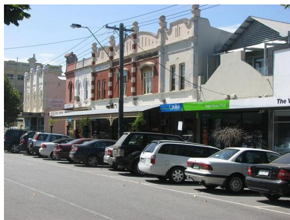
Figure 6.36-5 – The mixture of Victorian, Edwardian and Inter-war Shops along the south of Armstrong Street
