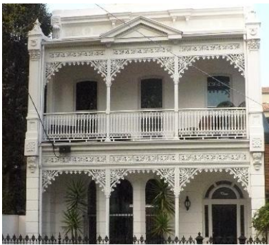
Figure 6.35-10 – Double-storey Victorian terrace house, Mary Street
