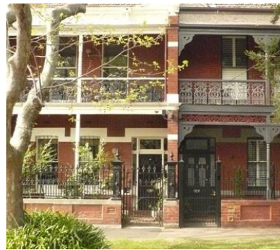
Figure 6.35-11 – Set of Double-storey terrace houses, Mary Street
