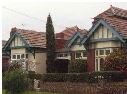
Figure 6.35–16 – Edwardian red brick villas, McGreggor Street
