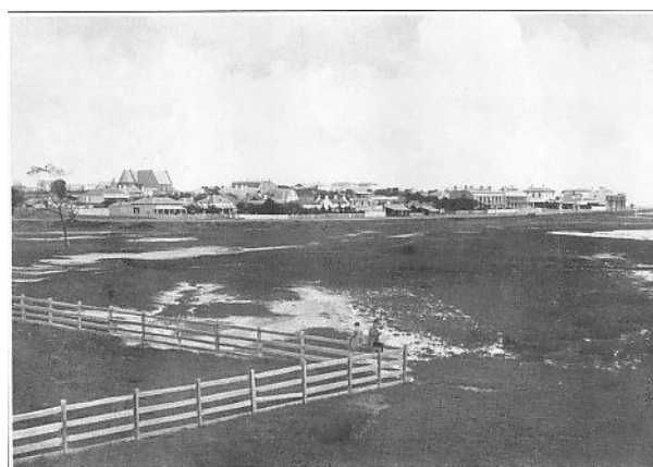
Figure 6.35-2 – A rare photograph of the WesternSwamp, c.1855, looking south-east towards Fitzroy Street, St Kilda
