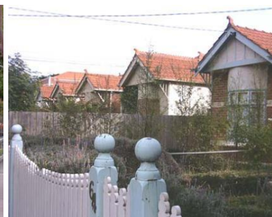
Figure 6.35-21 – Row of Edwardian red brick villas in Ruskin Street, Elwood
